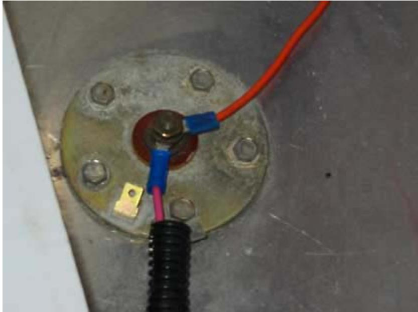
Now that all of the sensors have been installed and wiring run, its time to connect everything to the monitor. I found that while the panel is constructed pretty well, I suggest that you use a strain relief on the wiring near the panel.
